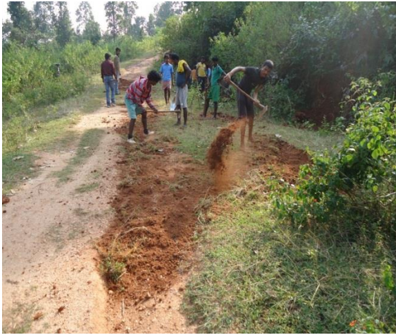
Village road construction by shramdaan construction
