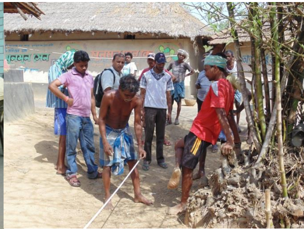
Construction planning in a plot donated by a villager
